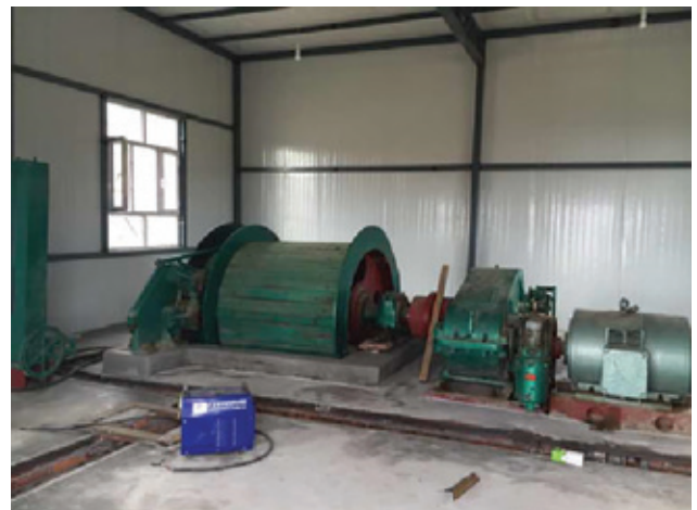
Winch system installment
